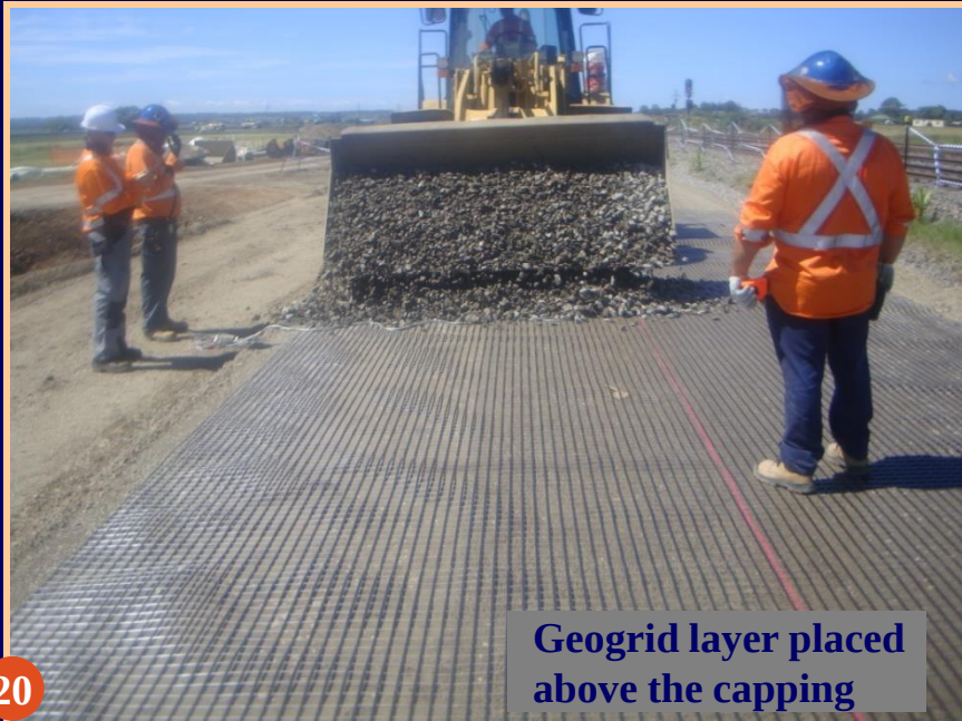
Geocomposite layer (geogrid+geotextile) before ballast placement
